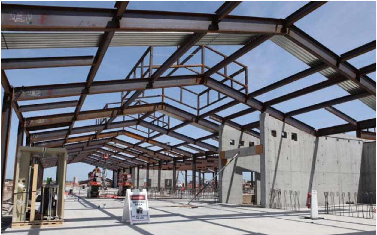
Construction work continues on the new Stockton medical facility.
