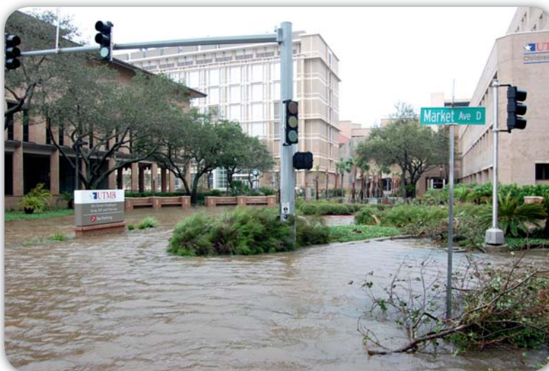
Flood waters destroyed the electrical and telecommunications systems of the hospital.
