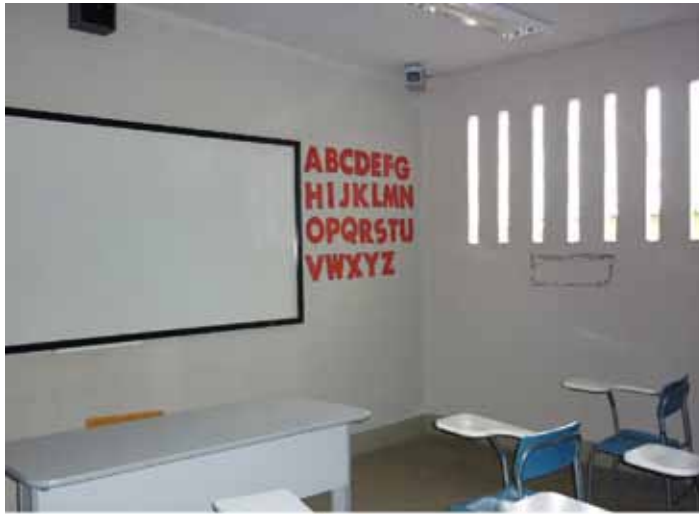
Window slits in classroom
