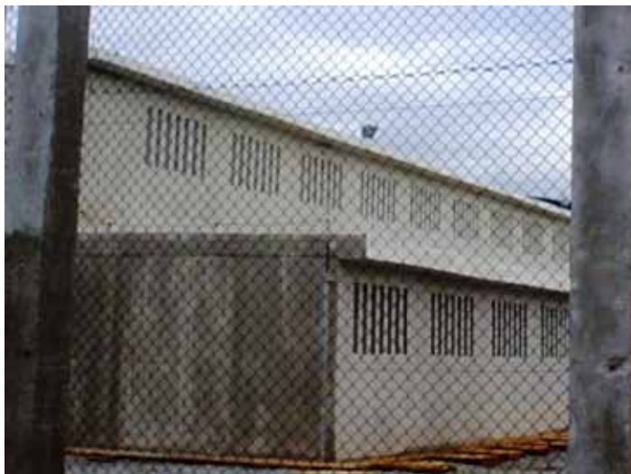
Window slits in cell pavilion
